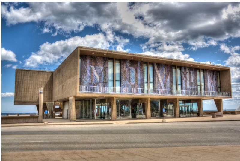
WMC on the shores of Lake Michigan, designed by architect Eero Saarinen
